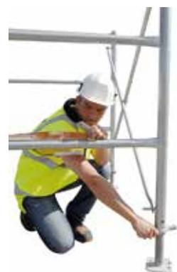
**5** Level the frame by turning the base jack.
