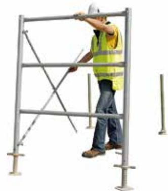
**2** Attach 2 diagonals at both sides of the frame.
